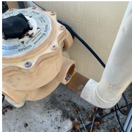
Amenity Center – Repaired back flow at splash pad – CBuss Before & After
