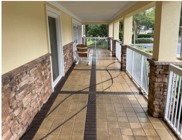
Amenity Center Pressure washed front patio of amenity center – GMS
