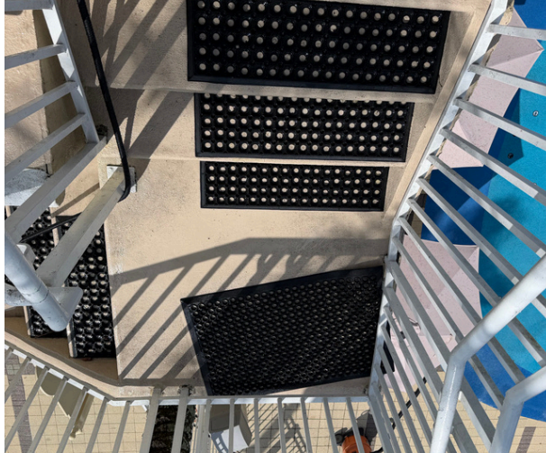
Amenity Center Pressure washed slide tower staircase –GMS
