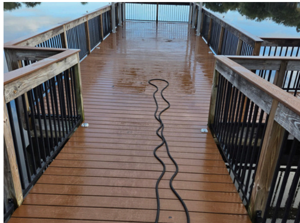
Amenity Center – Pressure washed lake gazebo dock – GMS
