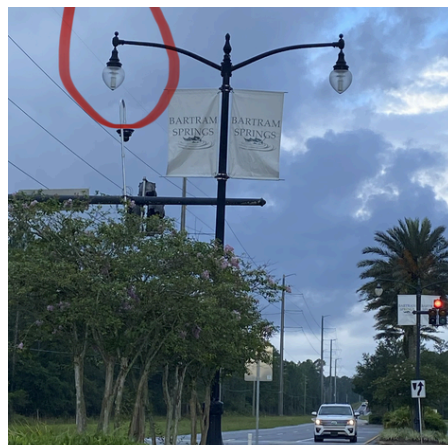
Bartram Springs Entrance - Repaired Lights on Race Track Road-Dobson Electric
