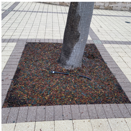
Amenity Center – Installed rubber mulch pool deck palm trees – GMS
