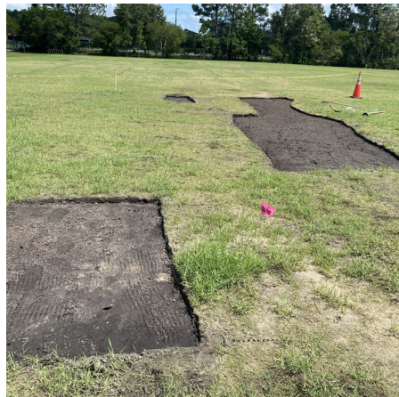
Veterans Park Field Repairs New Sod- Yellow Stone
