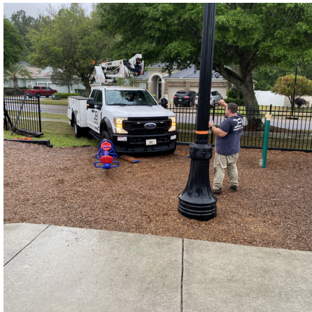
Amenity Center Took down damaged light pole - DEI
