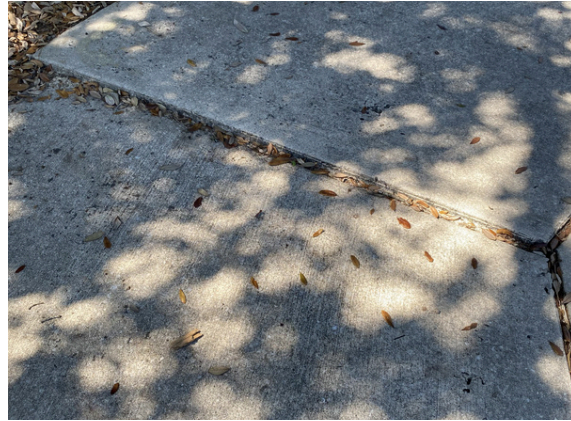
Amenity Center – Sidewalk Working on proposals – GMS
