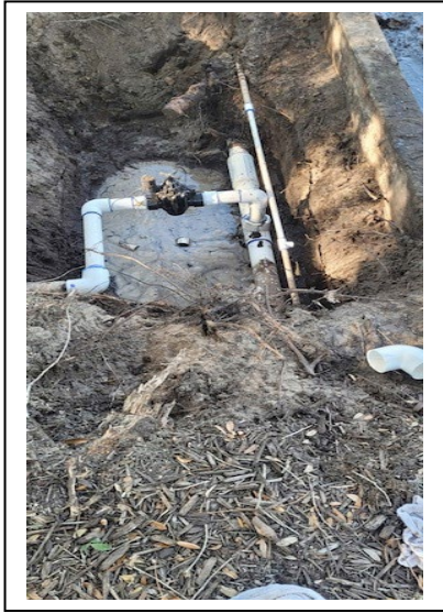
Irrigation Mainline Repairs- Cherry Lake Verde Go
