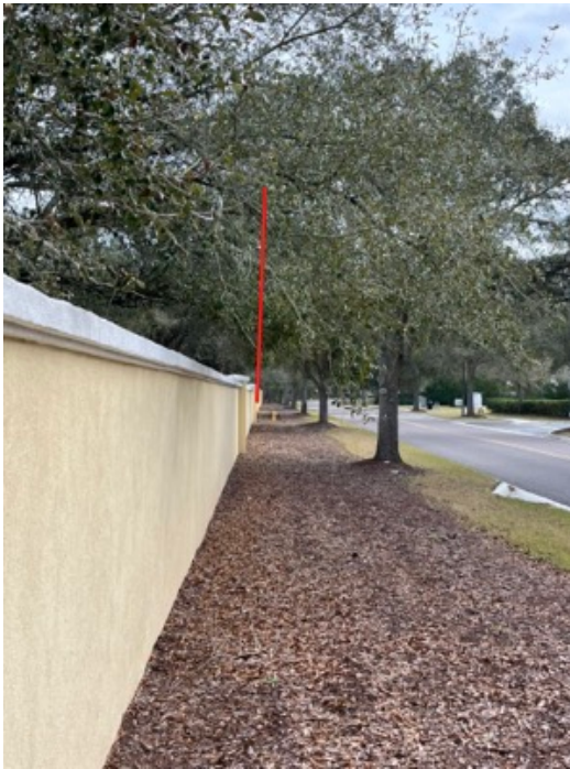
Area 6 - Across From Athletic Fields Assigned To Maintenance Crew Cut branches growing over the wall up to 10 feet for better wall clearance
