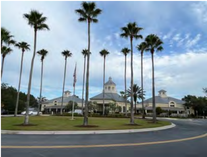
Area 1 Palm trimming was recently completed
