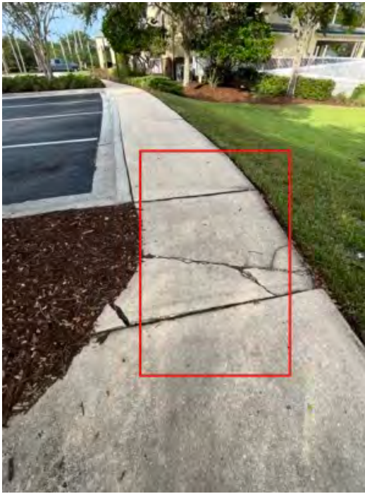
Area 8 Assigned To Safety Concern Markings on sidewalk are fading and can be resprayed and/or have sidewalks shaved
